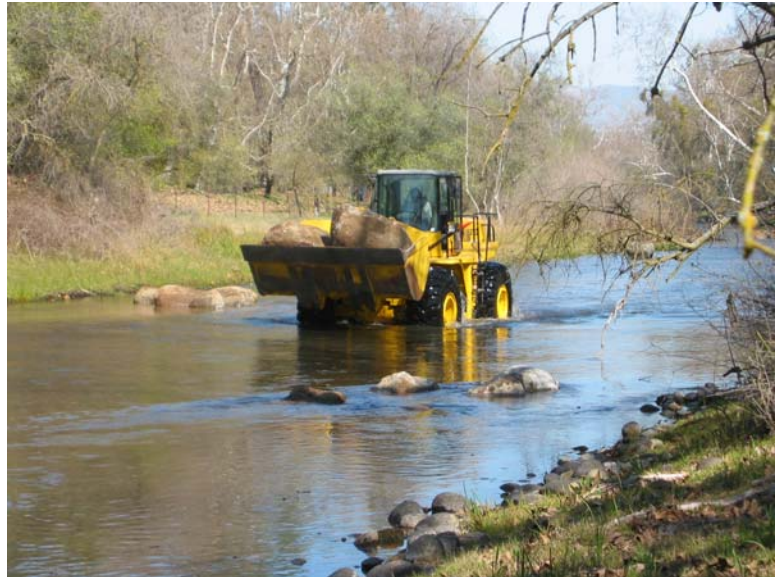
Figure 4-1. Placing boulders near Avocado Lake County Park
