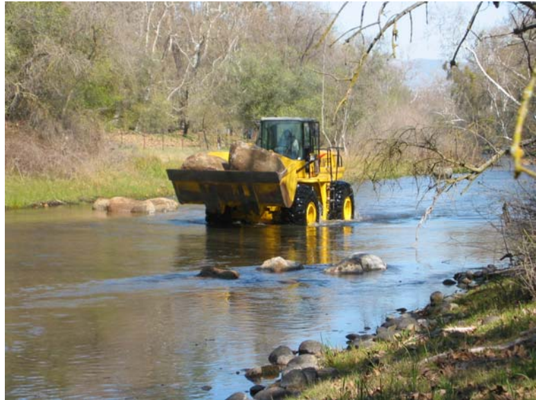
Figure 4-1. Placing boulders near Avocado Lake County Park
