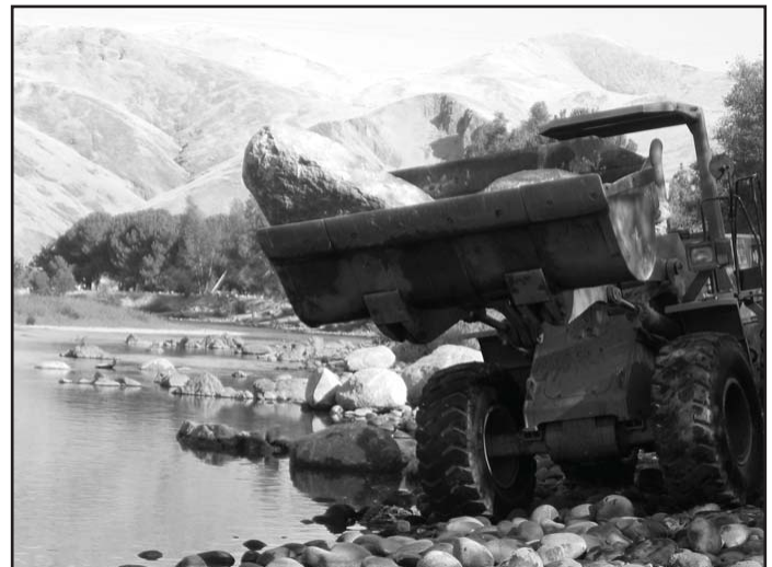
Boulders placed in the river improve habitat by providing shelter from flows for fish.
