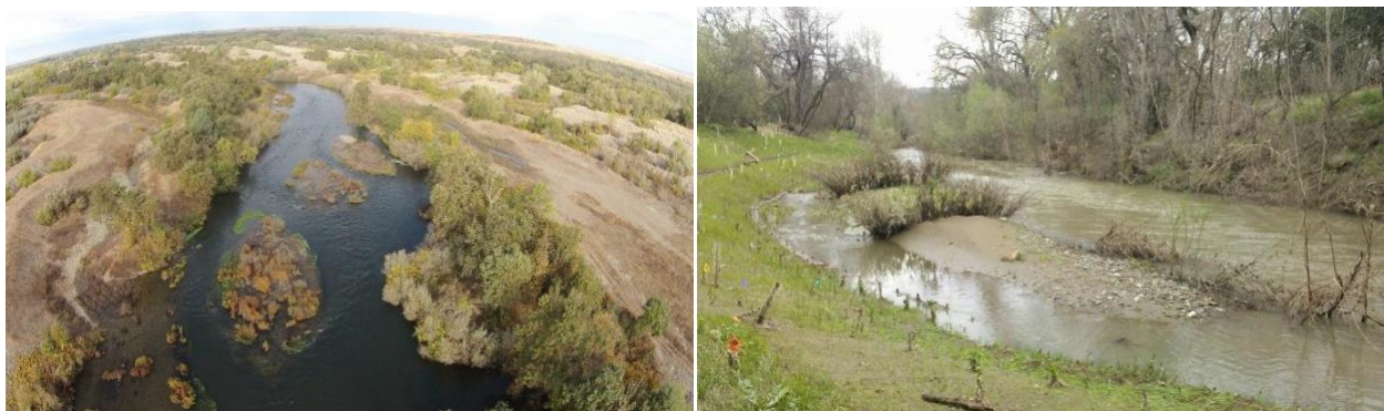
Figure 50. Example of constructed river islands. The left photo illustrates river island creation from the augmentation of spawning gravels on the Merced River, Ca. The right photo illustrates river island creation by excavating a channel behind the existing bank on the Napa River, CA.
