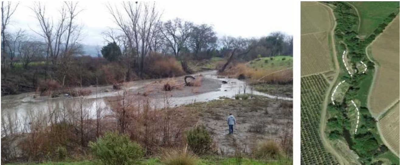
Figure 49. Example of local widening and gravel augmentation on the Napa River, CA. The left shows a photograph of gravel deposition at a local widening zone. The right image shows where local bank widening occurred at existing riffles. Left image is by author and right image from Google Earth.
