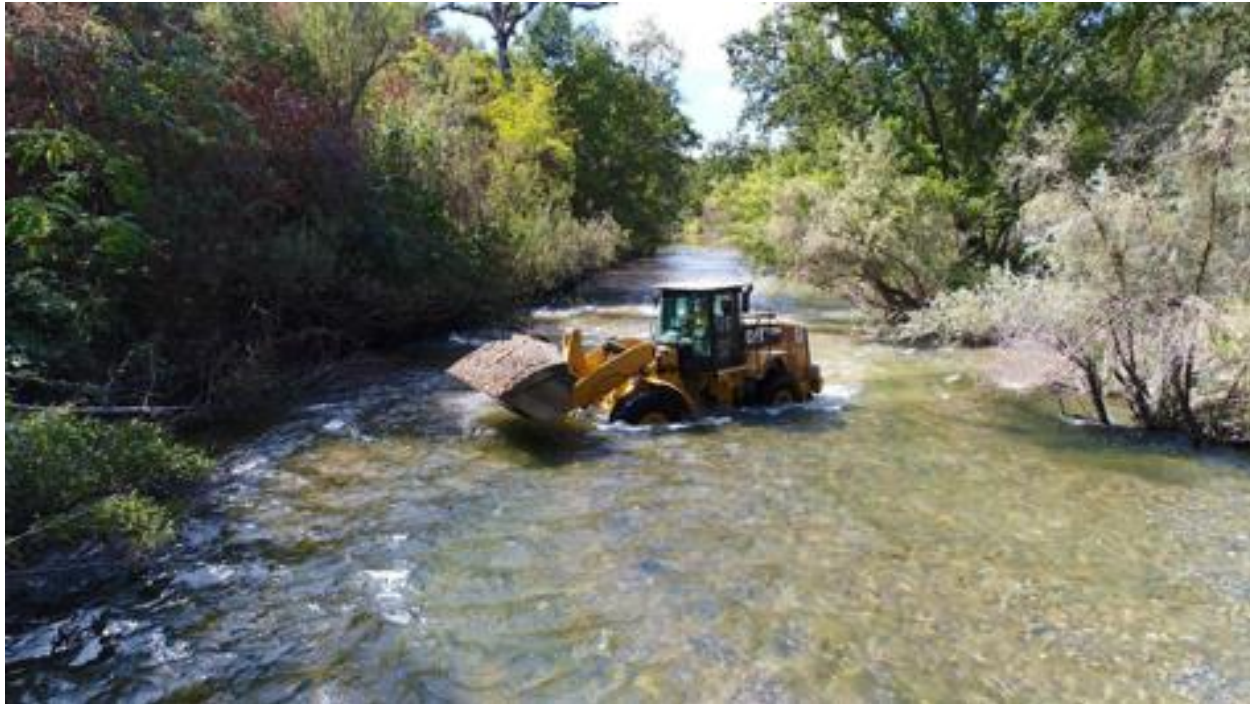
Figure 48. Example of riffle augmentation on the Stanislaus River, CA. The front-end loader is placing spawning gravels for Chinook Salmon and O. mykiss over an existing riffle where oversized substrate reduced spawning habitat conditions.
