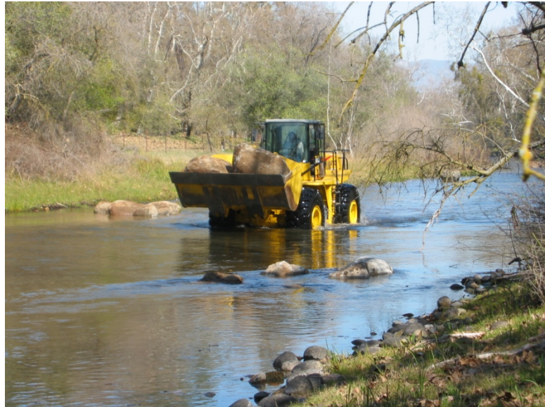
Figure 4-1. Placing boulders near Avocado Lake County Park
